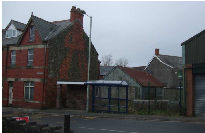
Figure 2 – Photograph of the application site (front)
